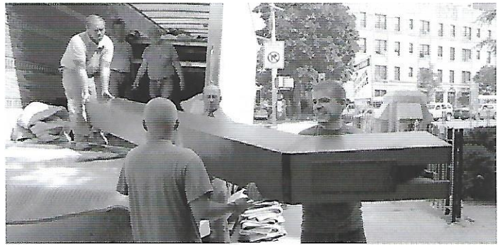
Photos of the largest pipe in the organ being taken off the truck and finally placed on its windchest inside the organ.
