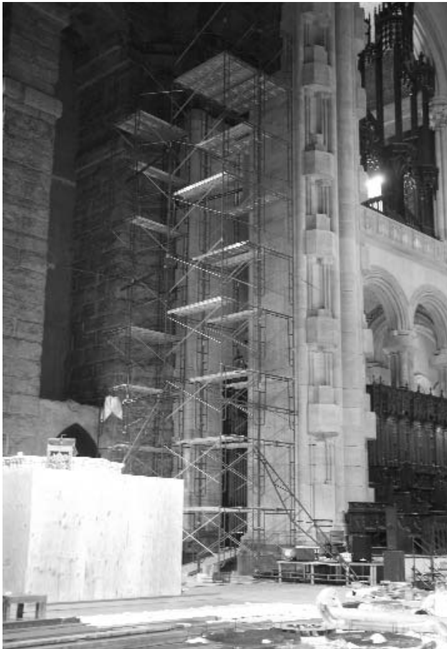
Scaffolding to the North Chamber
