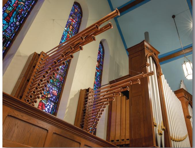
The new 8' Trompette-en-Chamade, with vertically oriented chests, and close-up view of new casework and facade pipes on the right side, in front of the Great and Solo divisions.
